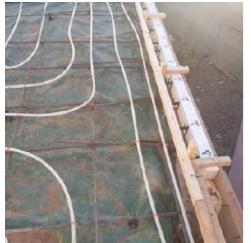
[EPS Insulation below slabs (R-10 min), at slab edges (R-20 min), at conc. stem and basement walls]
