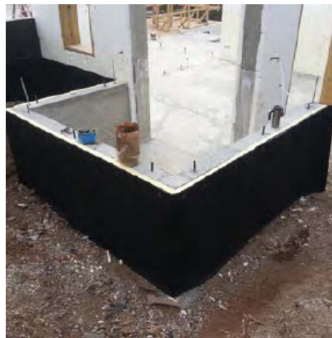
[EPS Insulation below slabs (R-10 min), at slab edges (R-20 min), at conc. stem and basement walls]
