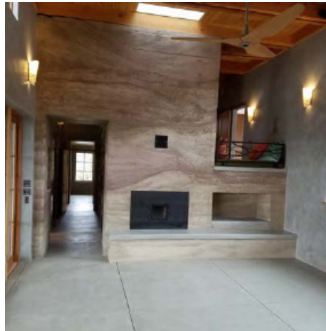
[Rammed Earth Masonry Heater w/ gasketed metal doors and flue to roof with exterior make-up air]
