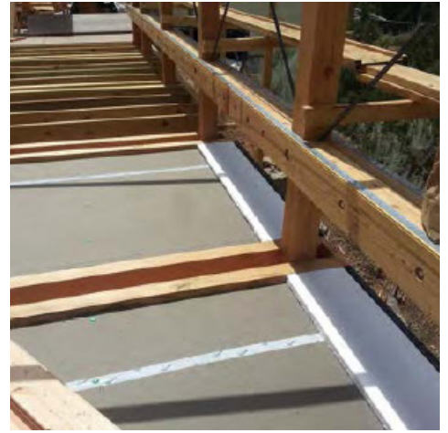
[Exterior polyisocyanurate wrap (2" at walls, 3 1/2" at roofs, 7" at dining room / bridge floor cavity)]
