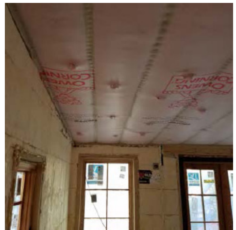
Full-cavity blown fiberglass insulation at all wood-framed walls (R-28 min) and roofs (R-38 min)]
