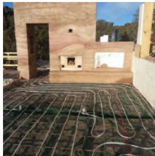
[EPS Insulation below slabs (R-10 min), at slab edges (R-20 min), at conc. stem and basement walls]
