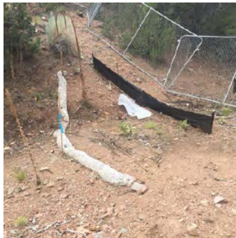
[Straw wattles filter / slow stormwater runoff]
