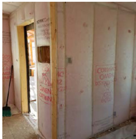
Full-cavity blown fiberglass insulation at all wood-framed walls (R-28 min) and roofs (R-38 min)]
