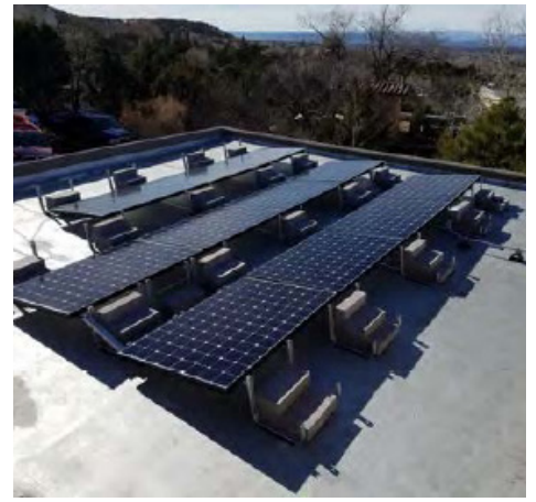
[6.7kW Roof-top photovoltaic array – prep for future battery backup / off-grid arrangement]
