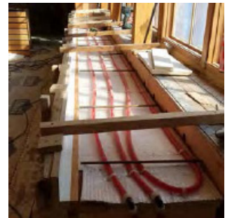
[EPS Insulation below slabs (R-10 min), at slab edges (R-20 min), at conc. stem and basement walls]
