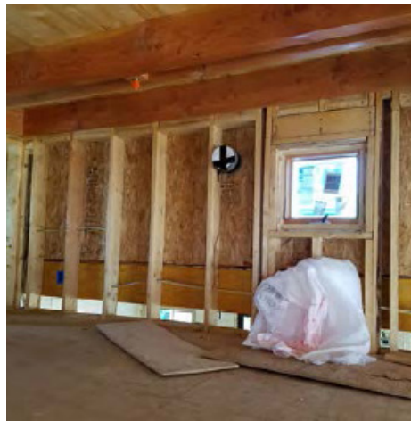
[4-pairs of Lunos HRVs (heat-recovery ventilators) – decentralized, balanced & quiet ductless, system]
