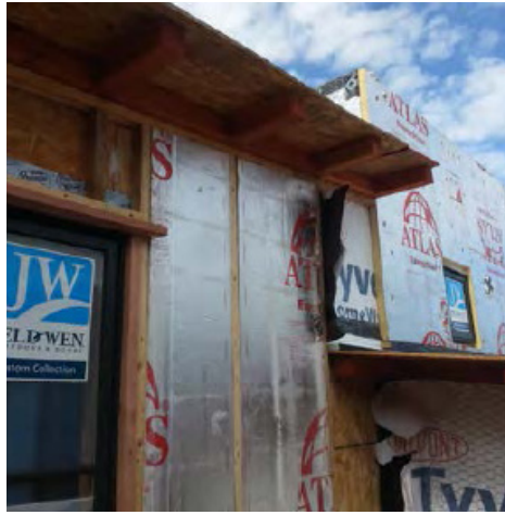
[Exterior polyisocyanurate wrap (2" at walls, 3 1/2" at roofs, 7" at dining room / bridge floor cavity)]
