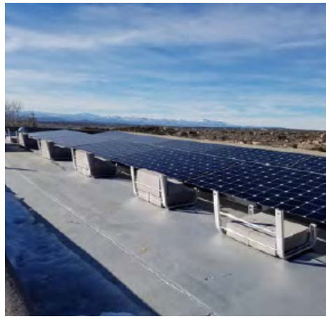
[6.7kW Roof-top photovoltaic array – prep for future battery backup / off-grid arrangement]
